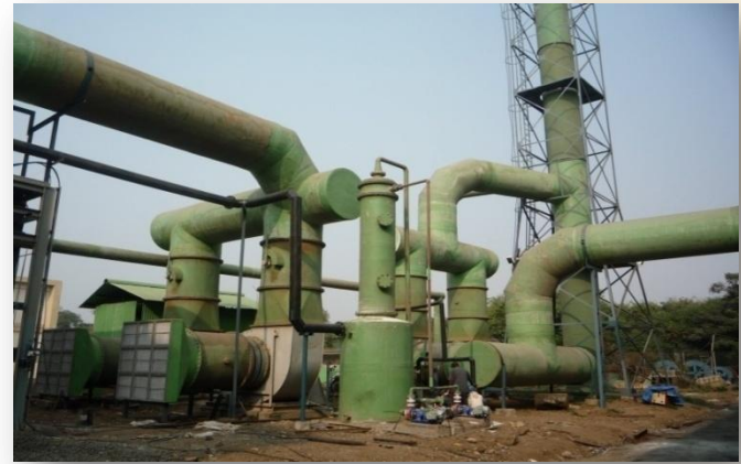
100000 m 3 /hr PP/FRP Ventillation System
